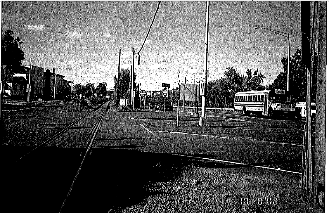
VIEW LOOKING: NORTH DESCRIPTION: WASHINGTON STREET INTERSECTION WITH ROUTE 9 SOUTHBOUND
