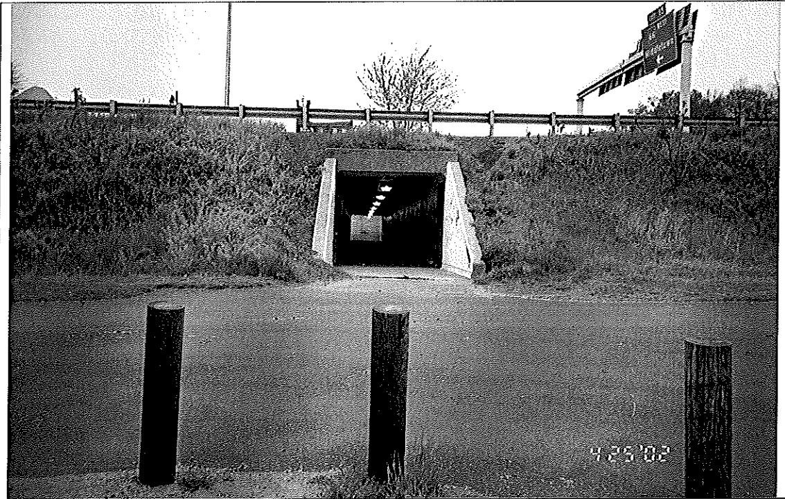
VIEW LOOKING: WEST DESCRIPTION: HARBOR PARK PEDESTRIAN TUNNEL UNDER ROUTE 9
