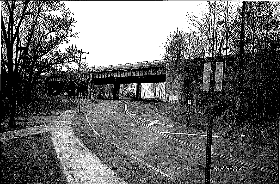
VIEW LOOKING: WEST DESCRIPTION: UNION STREET ROUTE 9 OVERPASS
