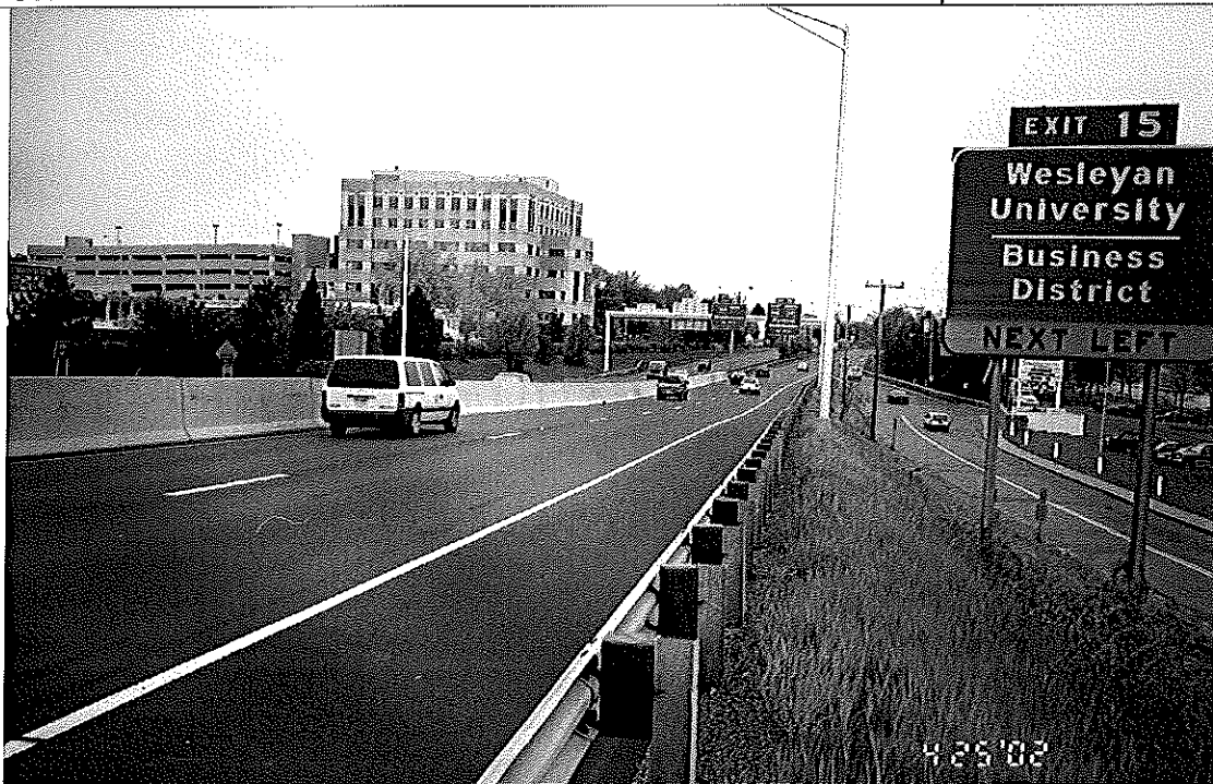
VIEW LOOKING: NORTH DESCRIPTION: ACCESS TO ROUTE 9 FROM UNION STREET UNDERPASS
